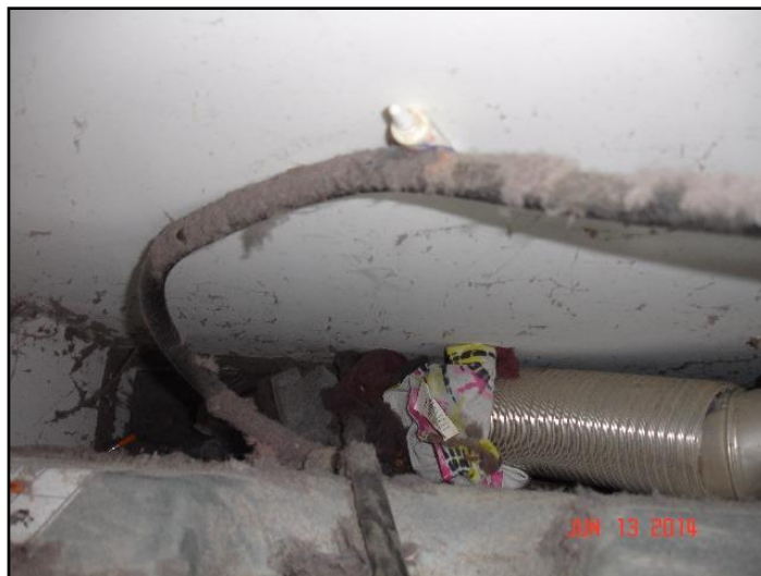
11. Rear of Dryer
