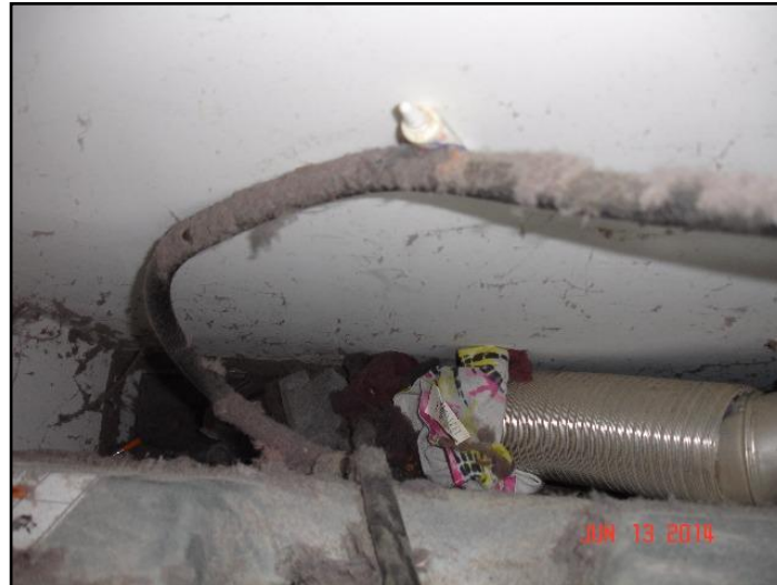
56. Rear of Dryer
