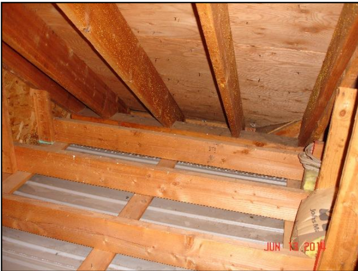
27. Rafters/roof joists
